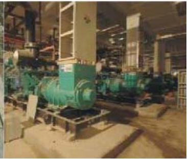
Basement Facilities - Infospace, Kolkata
