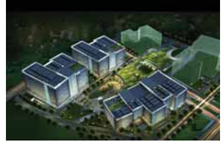
Infospace, Dundaheera, Gurgaon (G2-IST)
