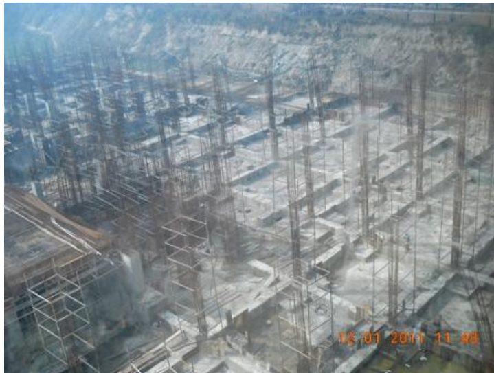
Phase II – work in progress
