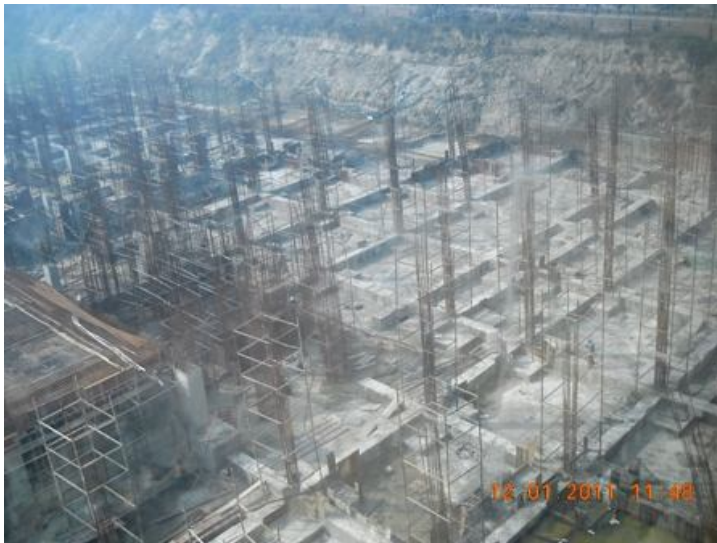
Phase II – work in progress
